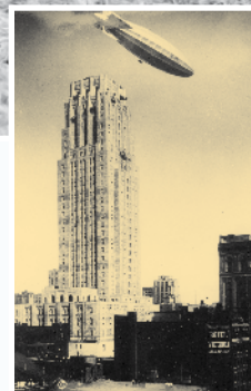
HIS MAJESTY KING GEORGE V'S AIRSHIP. "THE R-100" VISITED CANADA IN 1930 AND FLEW PAST COMMERCE COURT NORTH WHILE THE BUILDING WAS STILL UNDER CONSTRUCTION.
