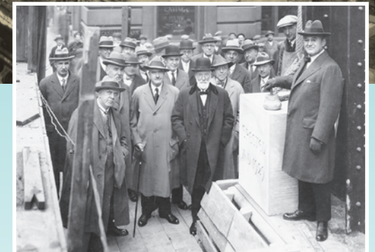
SIR JOSEPH FLAVELLE LAYING THE CORNERSTONE, 1929
